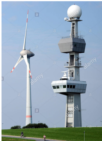
(a) Meteo station (wind)
