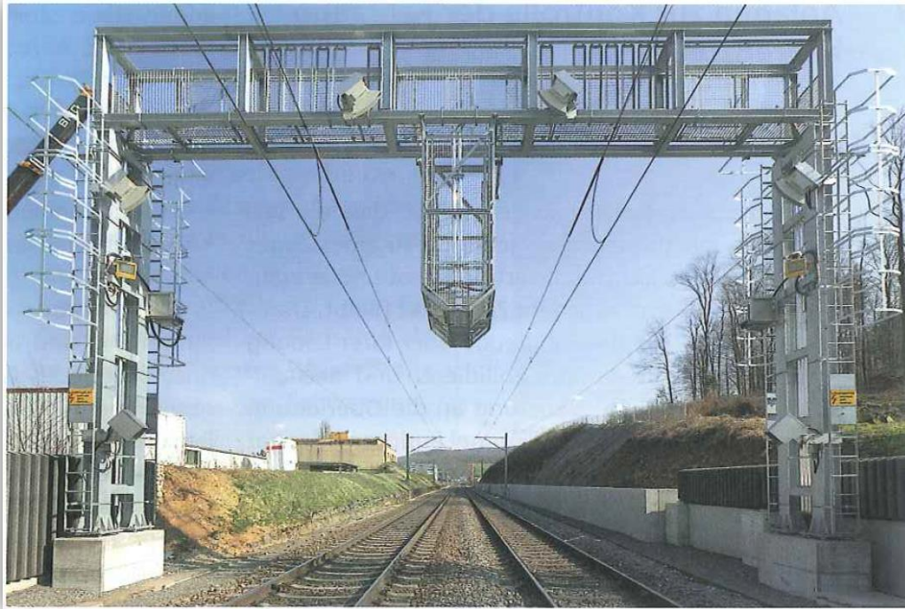
Gate controls in Switzerland (100 positions)
