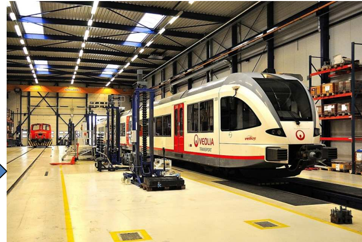
STADLER Maintenance Facility in Venlo
